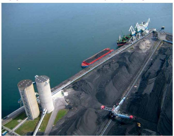
Coal is one of the biggest cargoes involved in dry cargo transshipment, and conveyor belt systems remain a highly effective method of transportation within storage and distribution areas. The belt itself is often the most vulnerable part of a conveyor system. Every time a conveyor has to be stopped means cost, not only in terms of the replacing and fitting the actual belt, but also in terms of lost production time.
