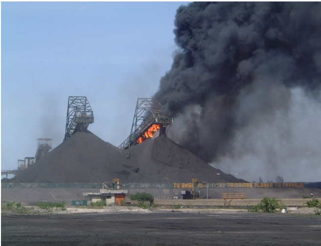
Figure 1. Coal conveyor fire.
