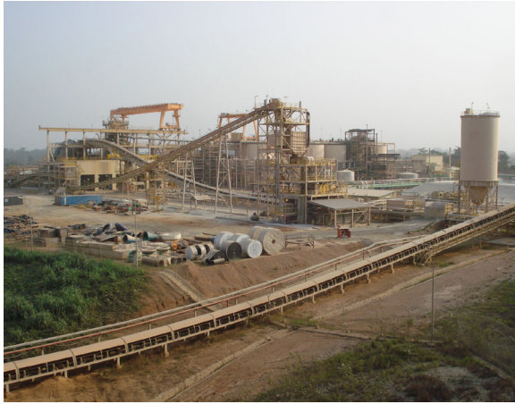
Conveyors are the most effective bulk handling method.
