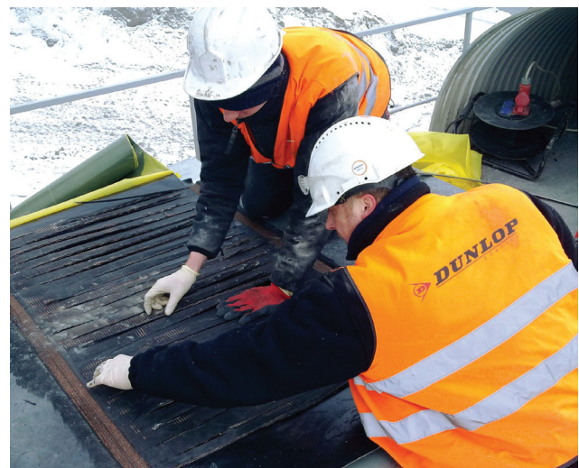
Using a finger splice can mean that a lower and less costly spec belt can be used.
