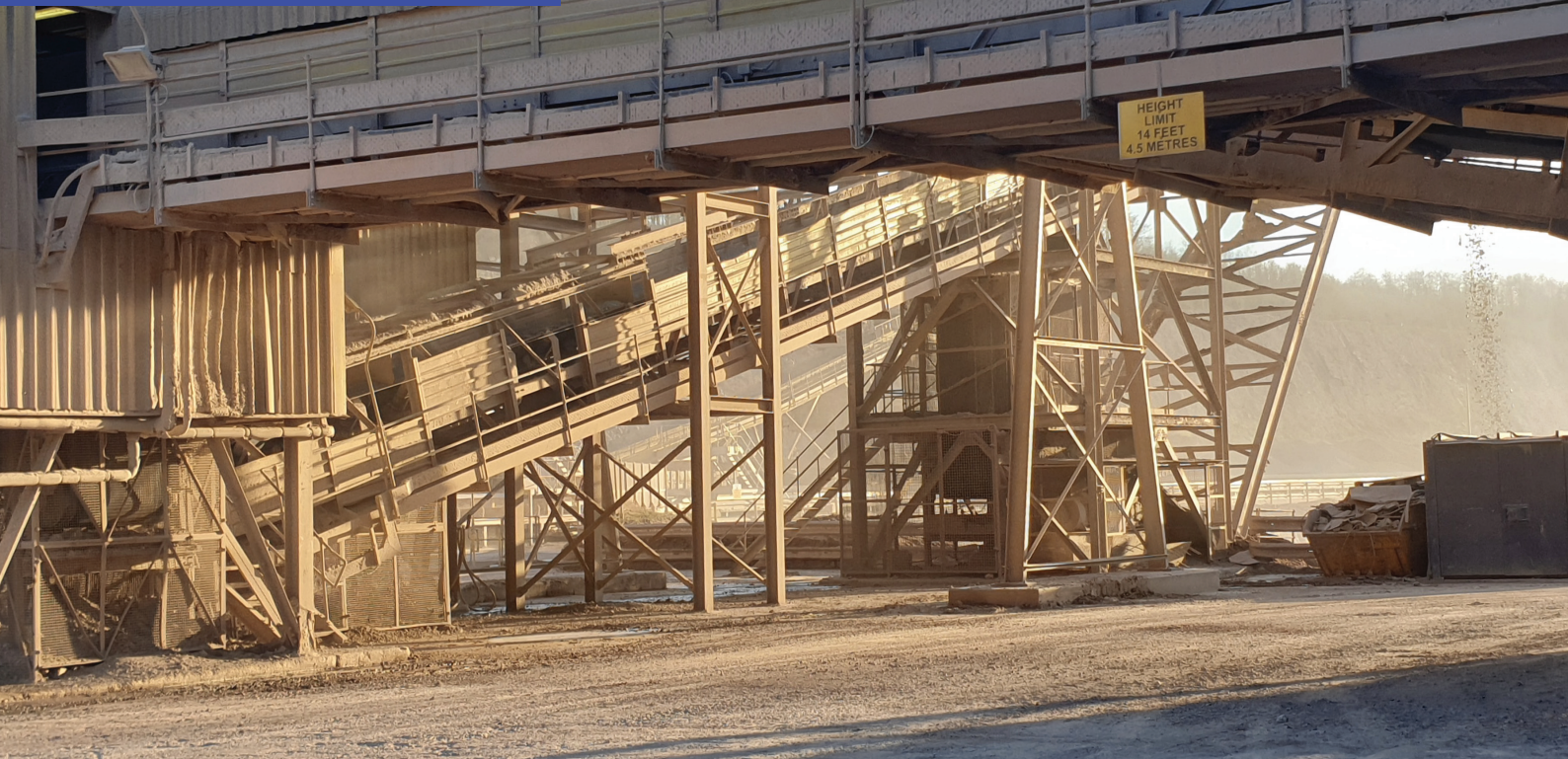
The C7 horizontal conveyor at Hanson's Whatley Quarry
