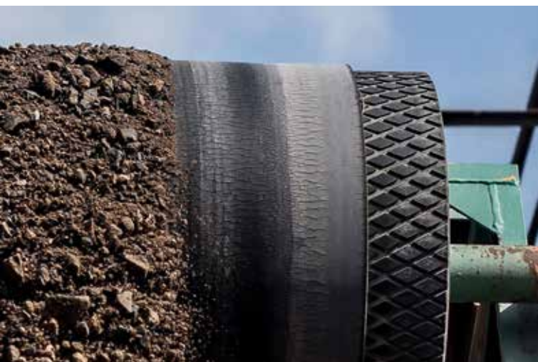
The first signs – small cracks appear on the surface of the rubber.
