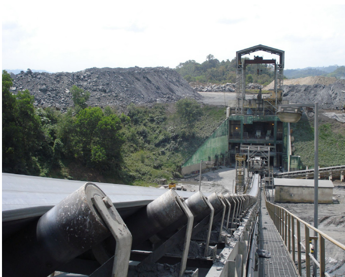
Bigger is not always better – installing a heavier belt can increase absorbed motor power.
