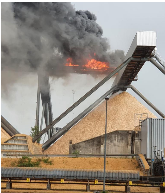
Conveyors convey fire extremely quickly – every second counts.
