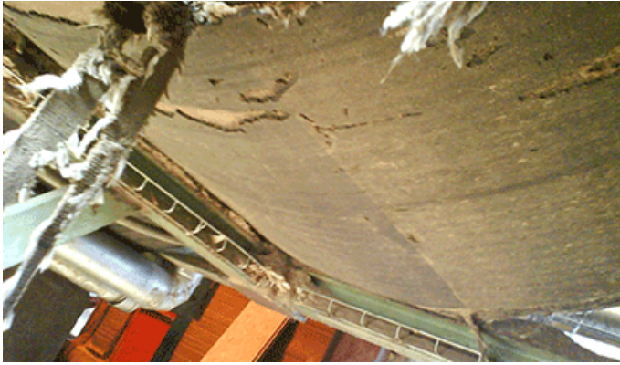
Photo courtesy of Dunlop A badly damaged conveyor belt
