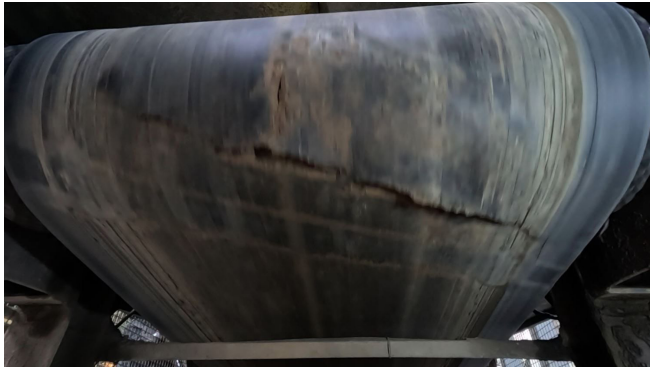
It is estimated that splice joint problems account for some 80% of unplanned stoppages.
