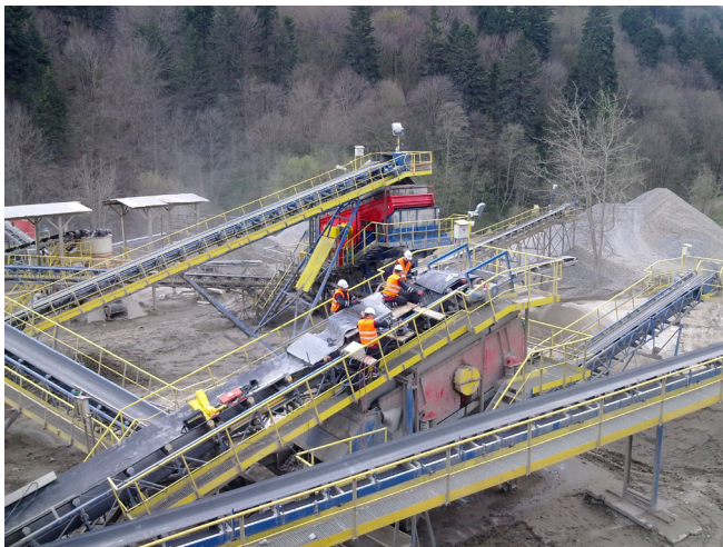
The cost of splice repairs and lost output is considerable.
