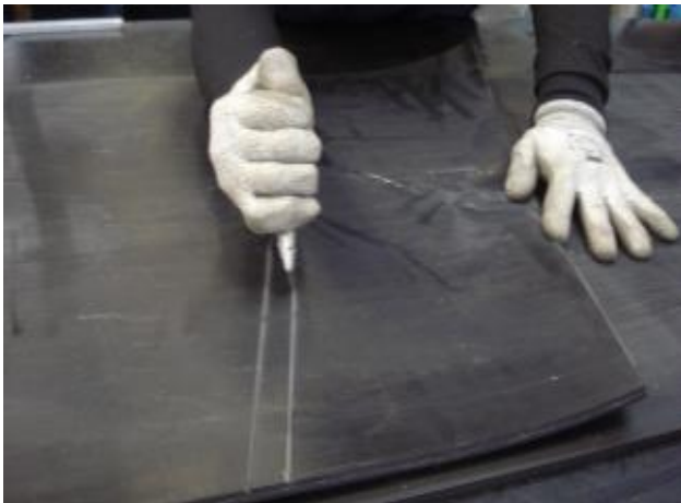
Photo 2. Cutting the filler strip
