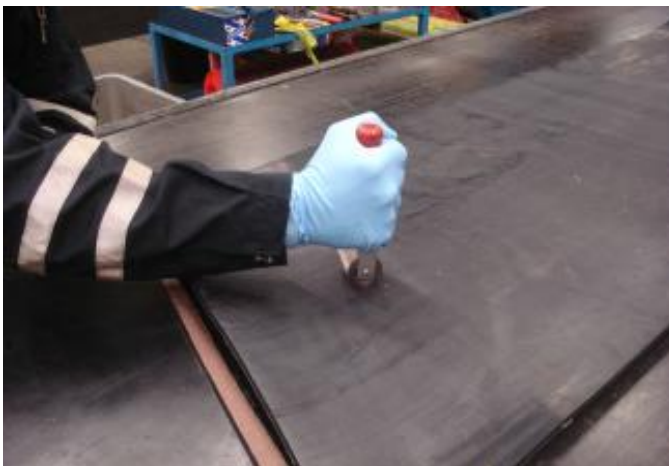
Photo 11. Roll the belt-ends together
