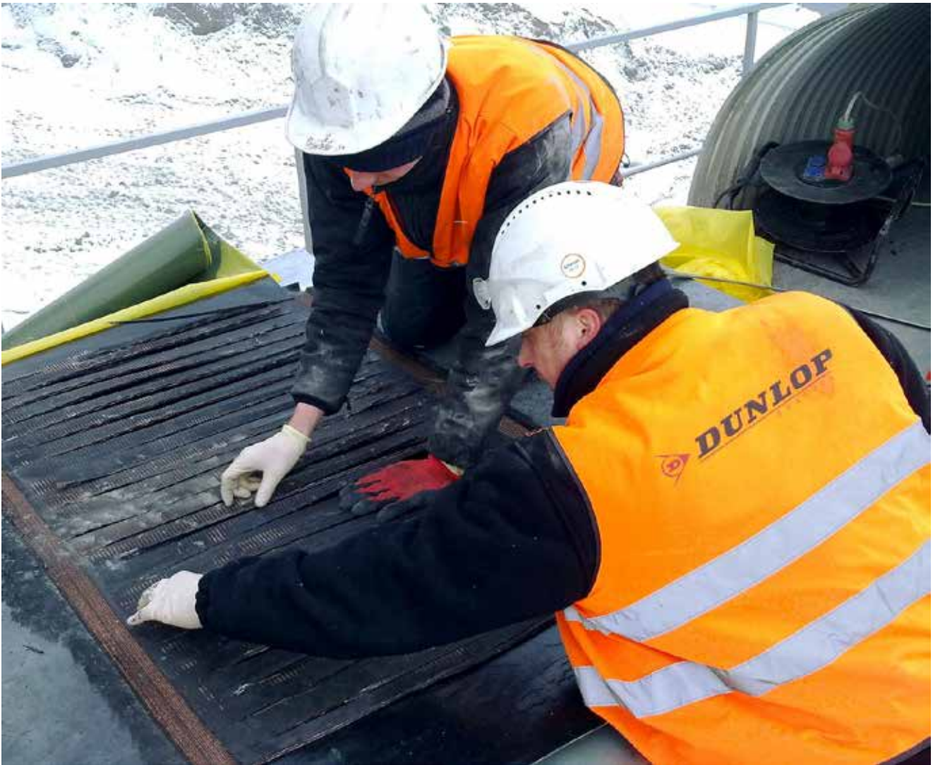
Finger splices are far stronger and more reliable and retain a much higher tensile strength. (Image courtesy of Fenner Dunlop Conveyor Belting).
