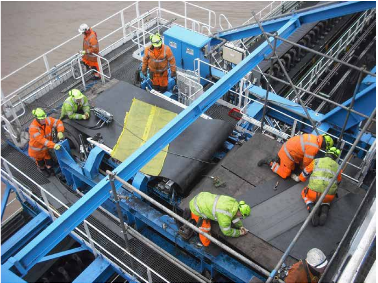
Splice joint problems are a major cause of stoppages for repair or replacement.
