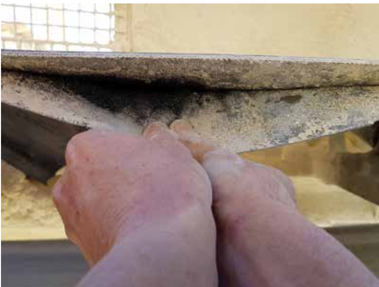
Insufficient elongation can cause delamination.
