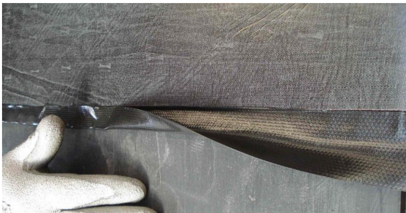
Photo 18: Applying second skim layer next to fabric
