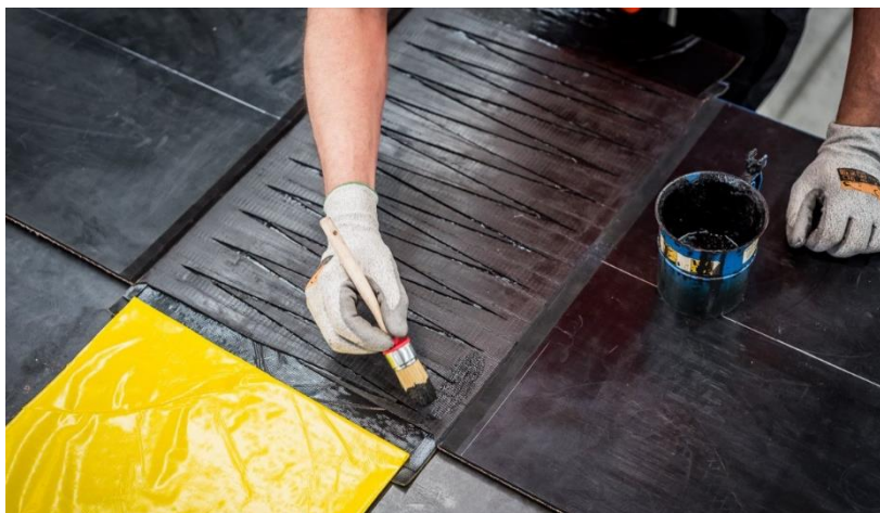
Photo 21: Solution on top of fingers
