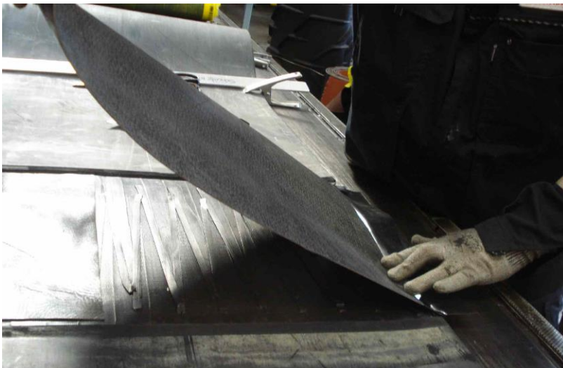
Photo 24: Wrap fabric around the carcass
