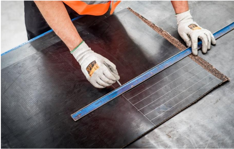
Photo 4: Drawing the finger widths
