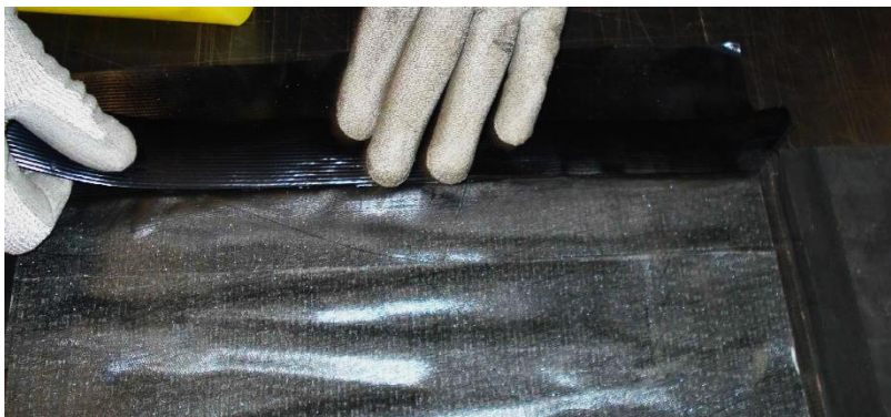
Photo 29: Applying rubber edges
