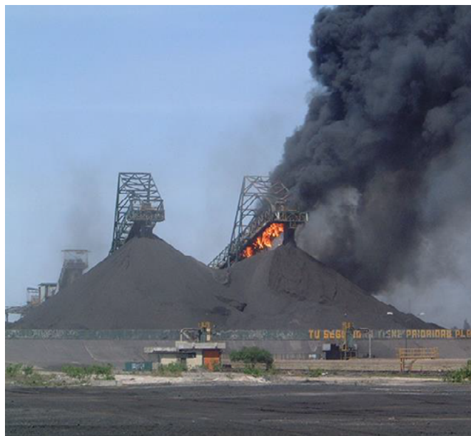
No conveyor belt is fire proof
