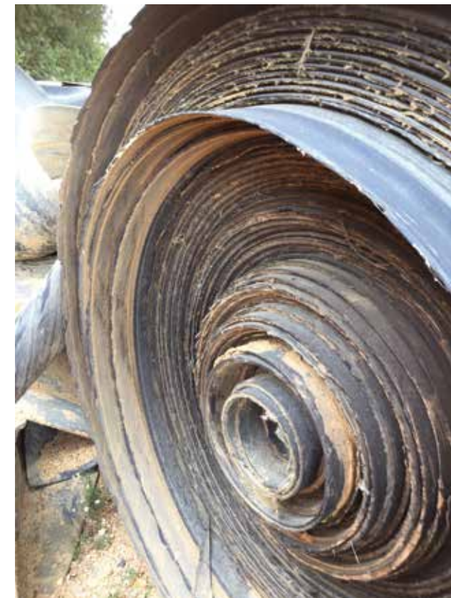
Misaligned multi-ply belts are quickly damaged when they hit the framework of the conveyor.
