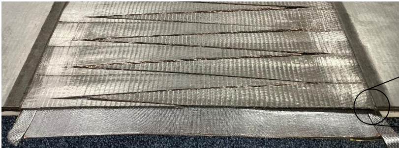
Photo 22: Correct position of the bottom cover
