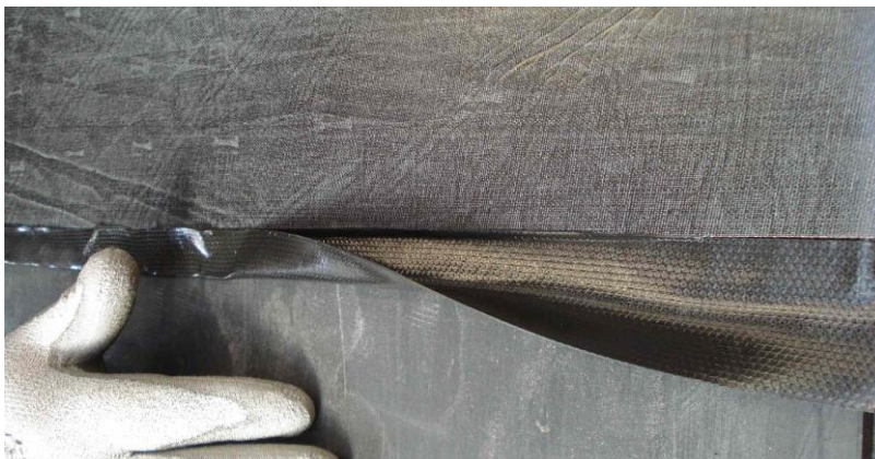
Photo 18: Applying second skim layer next to fabric
