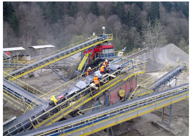
Figure 4. The cost of splice repairs and lost output is considerable
