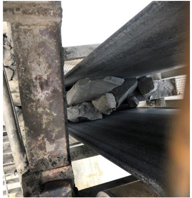
Figure 3. A big cause of stoppages is material becoming trapped.
